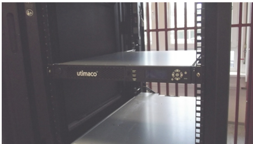
Figure 24 : Square style hole mounting posts
