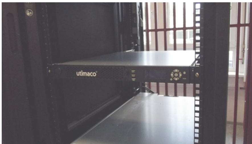
Figure 24 : Square style hole mounting posts
